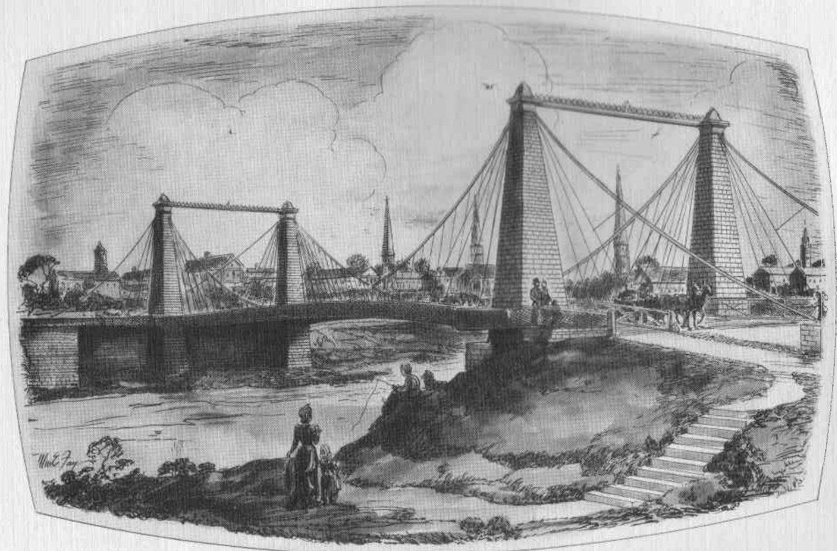
SUSPENSION BRIDGE, LOOKING EAST
