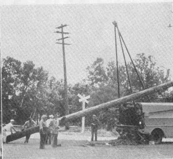
POLE SETTING CREW
