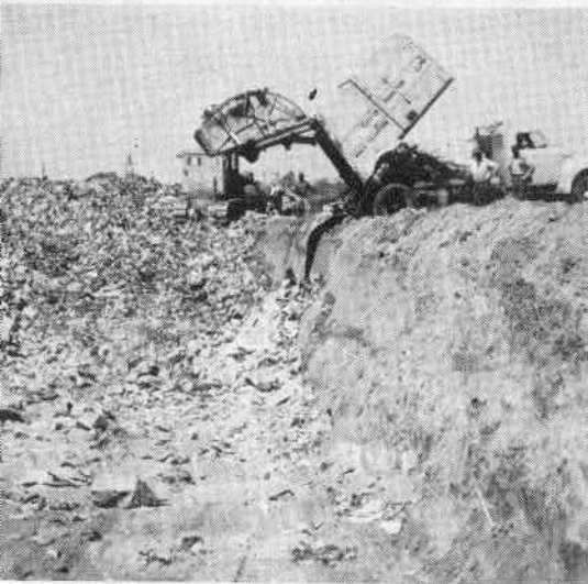
DUMPING INTO TRENCH
