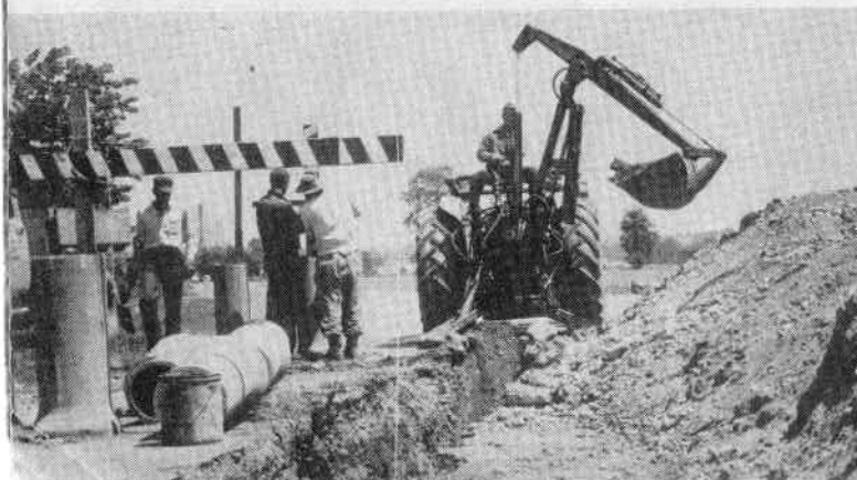
STORM SEWER INSTALLATION
