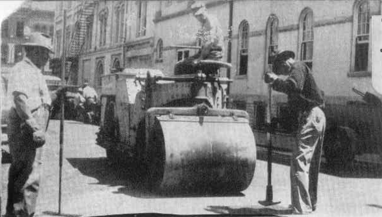
ROAD PATCHING CREW
