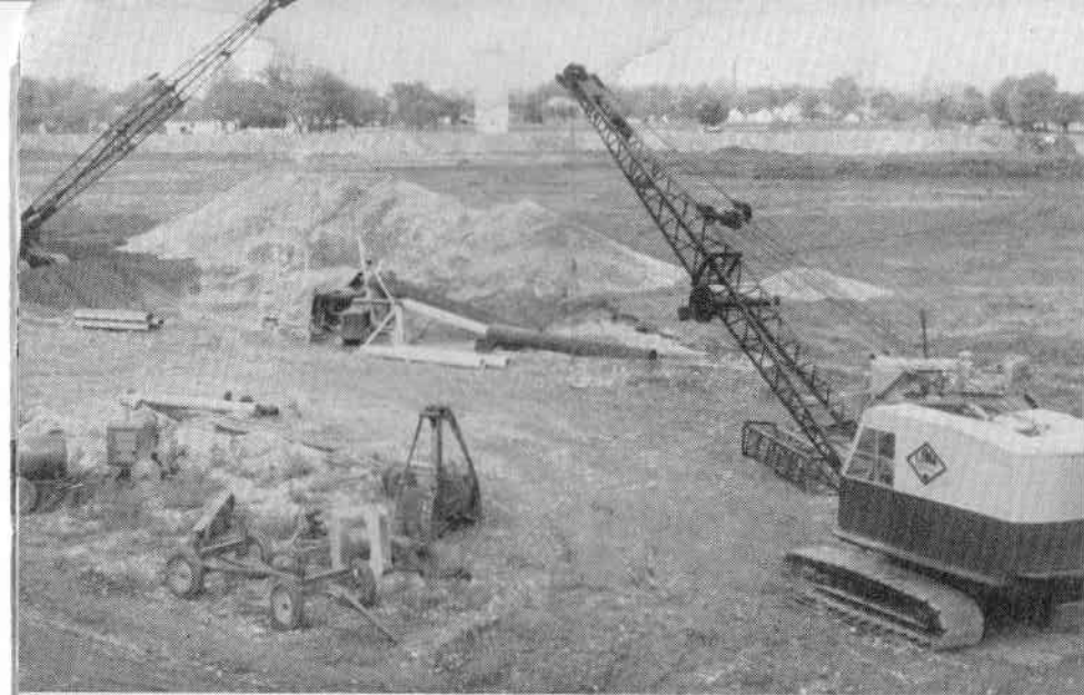
START OF WORK — MAY, 1954
