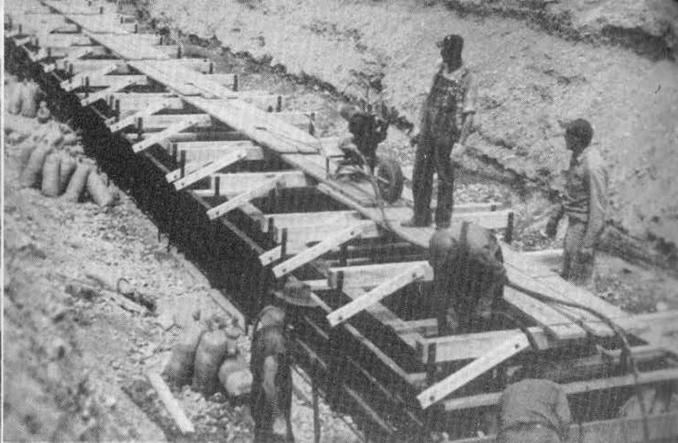
FORMS FOR CONCRETE PIPE LINE
