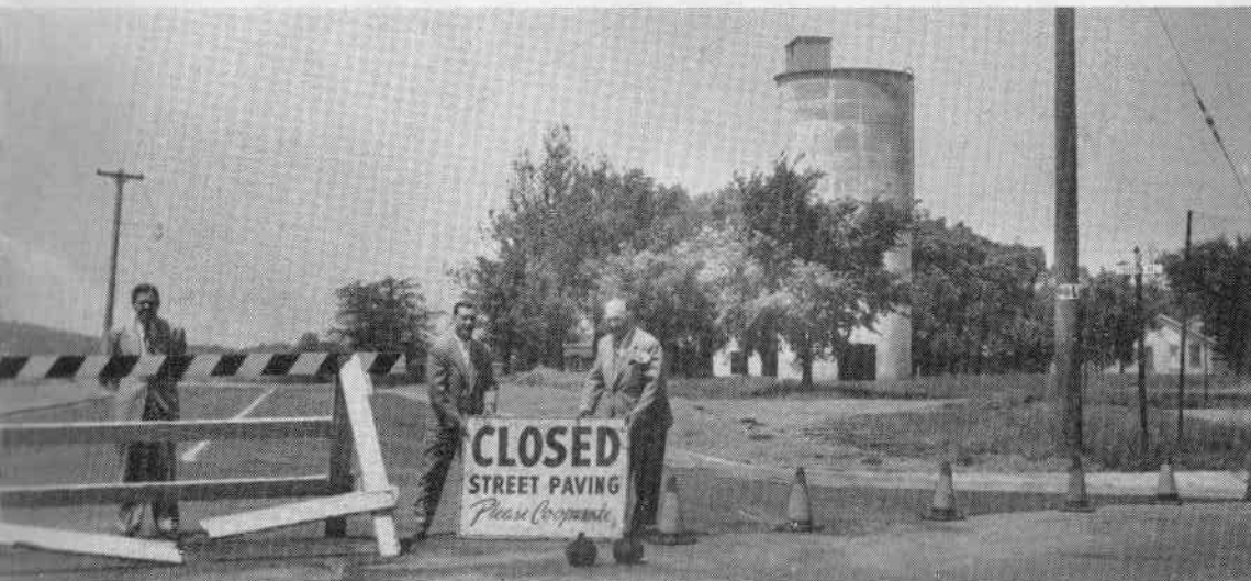
OPENING FINAL SECTION OF NEILAN BOULEVARD
