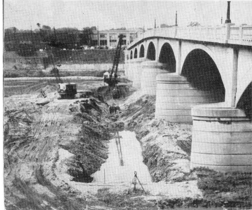
RIVER CROSSING AT BLACK STREET BRIDGE
