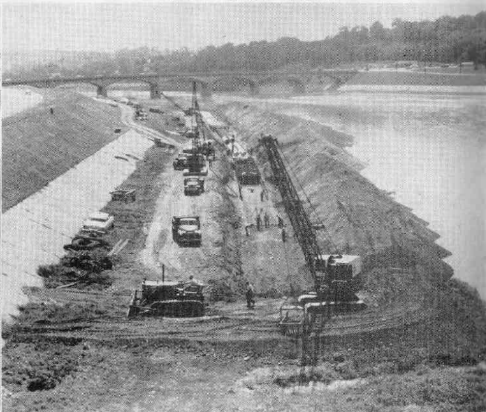
LOOKING SOUTH FROM RAILROAD BRIDGE
