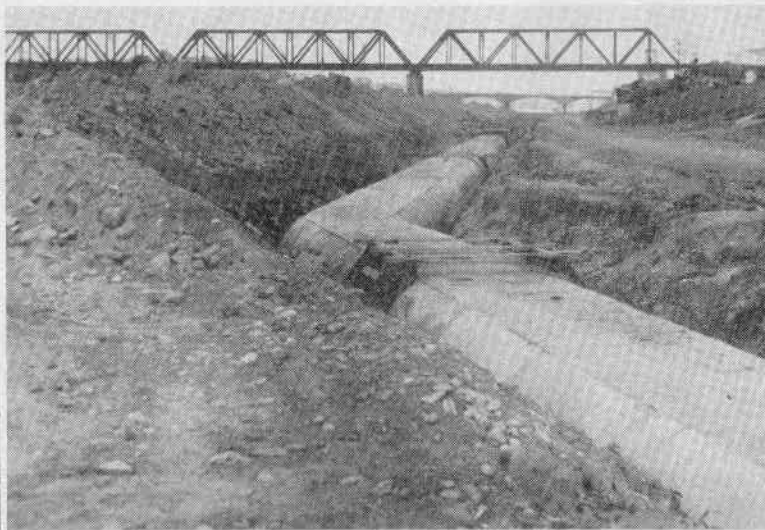
COMPLETED SEWER ENCASING 60" AND 48" PIPES
