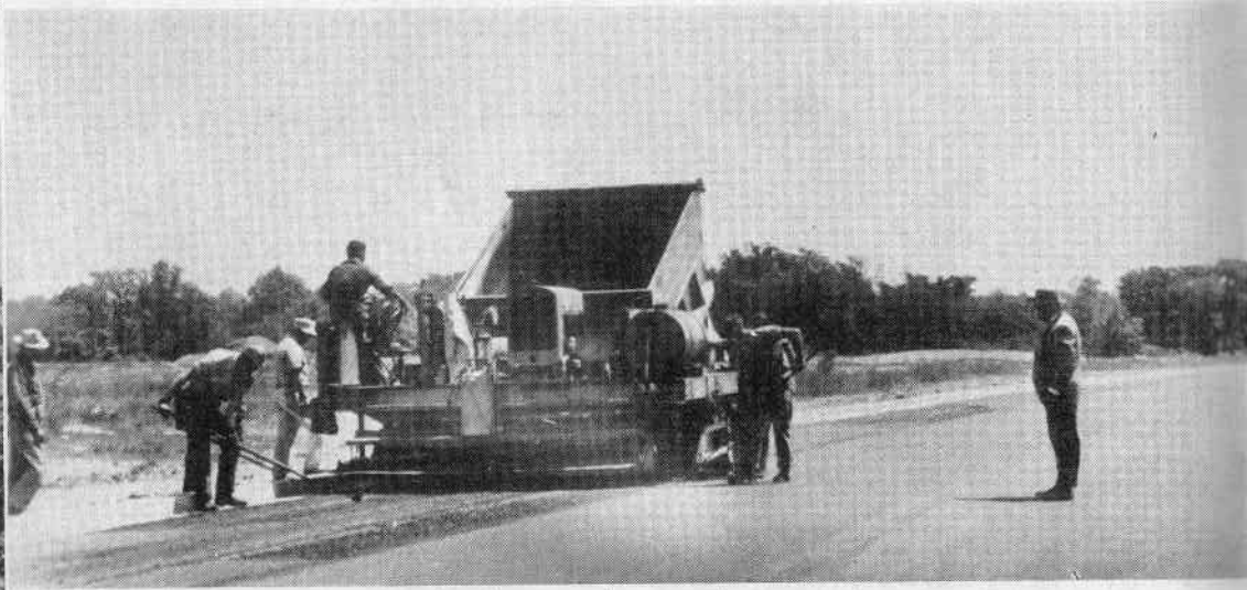
PAVING FINAL SECTION OF NEILAN BOULEVARD
