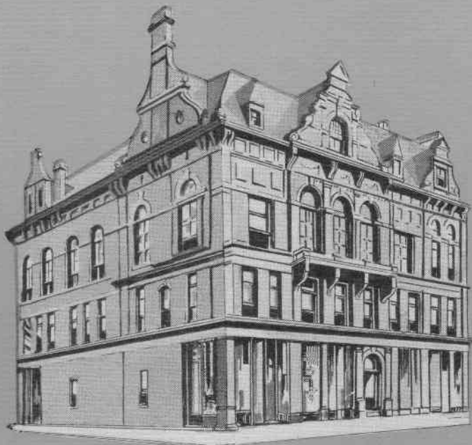
Second location of Home Federal—Reily Building: Hamilton, Ohio
