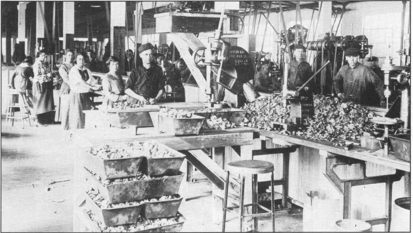
"Team Picture Day" 1920 style. These photos give a view of how we manufactured Casters in the early years. Machines were powered by the overhead line shafts which turned the belts. Most casters in that era were shipped in wooden barrels.
