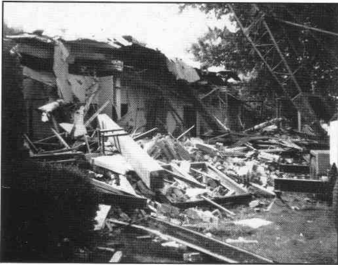
Demolition of the "old" office began in the summer of 1979.
