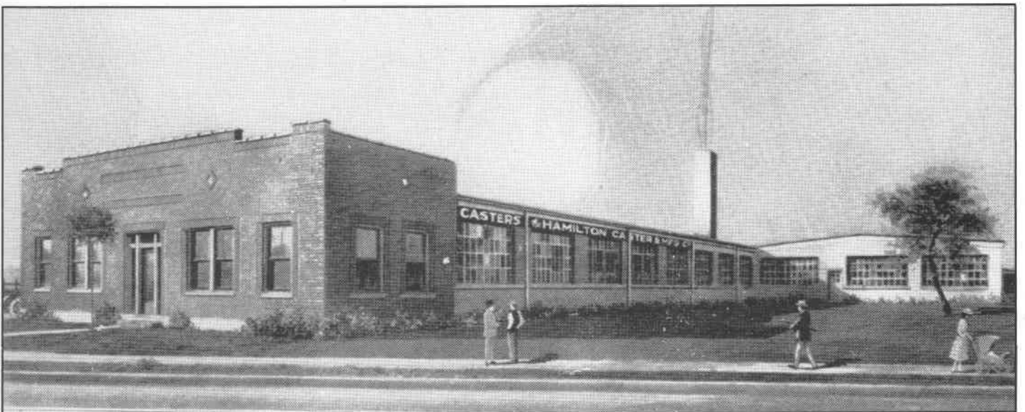
A 1920 view of the Dixie Highway facility. This building stood alone as our sole facility through most of the decade.
