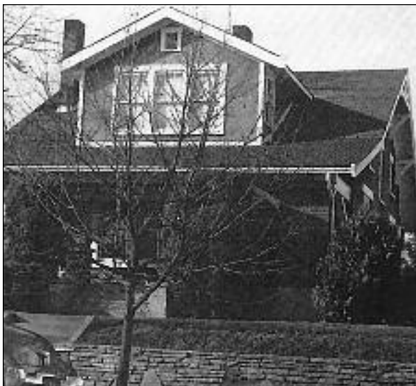
20 West Walnut Street
