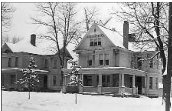
123, 129 West Walnut Street
