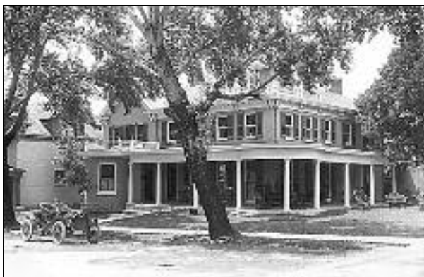
103 West Walnut Street
