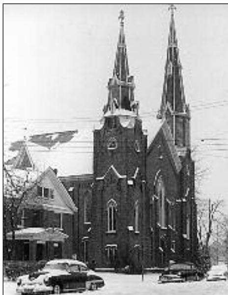
14 North Poplar Street
