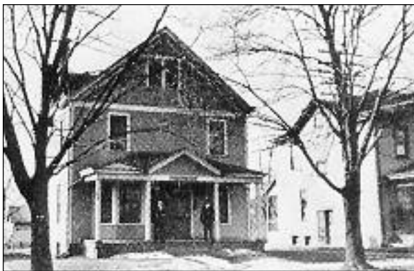
15, 17 West Walnut Street
