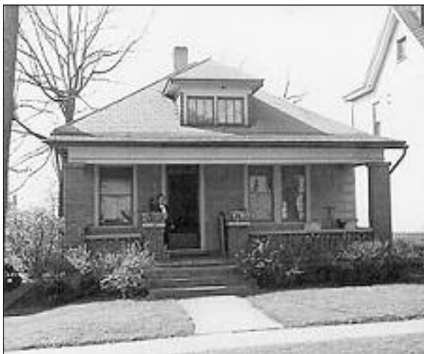
9 West Walnut Street
