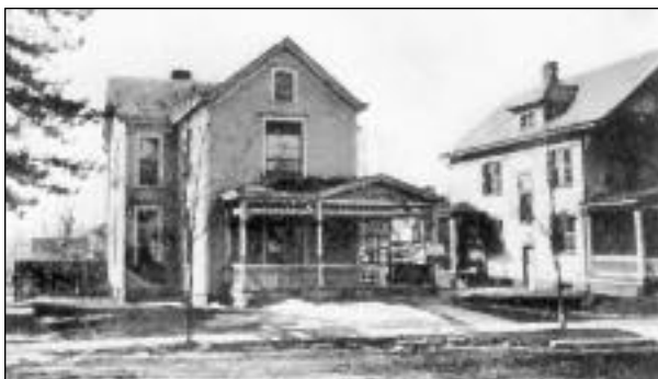
115, 117 West Walnut Street
